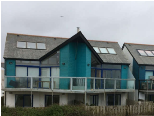
Use of non sustainable plastic cladding planks
