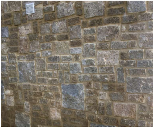
Out of local character layout of granite slips (too regular)
