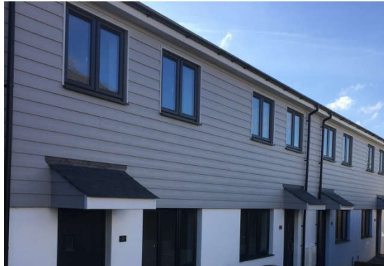
Use of non sustainable plastic cladding planks
